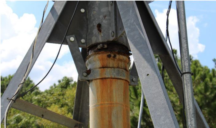
Figure 18. Sufficient greasing, proper connections, and bolt tightness are critical at the pivot point. Service and replace parts as necessary to ensure correct operation throughout the season.
